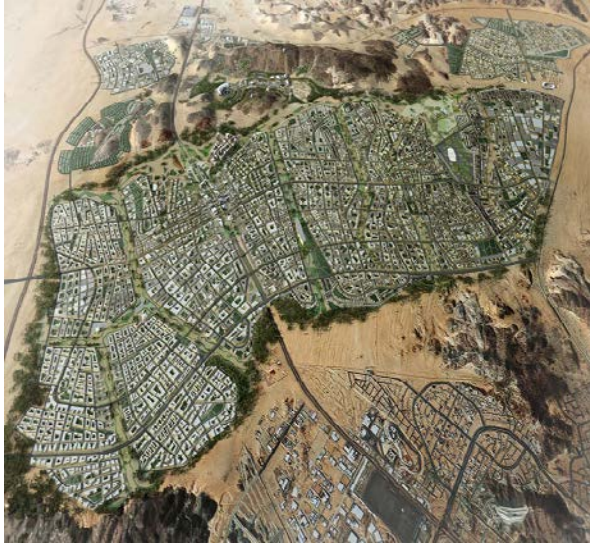
Figure C: The Project Site
